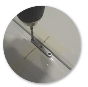
• Lightly mark position of outside holes of the mounting block in the roof channel.
